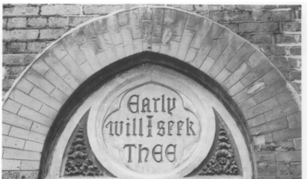
Architectural detail above School entrance
